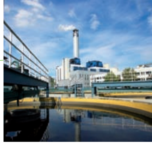
Ruhleben sewage sludge incineration plant
