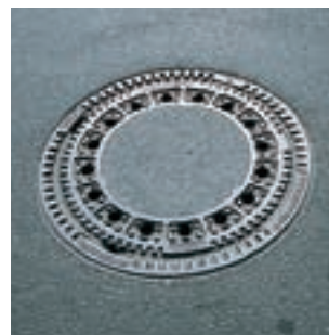
Manhole Each sewer has an opening to the surface every 60 meters or so. Through these openings, sewer workers can enter the sewers, bring in cleaning equipment, remove blockages and / or sewer sludge and repair damage.
