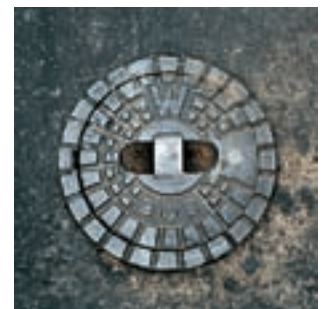
Slide valve fitting Found on roads or footpaths for shutting off pipes. The blue sign indicates their position.
