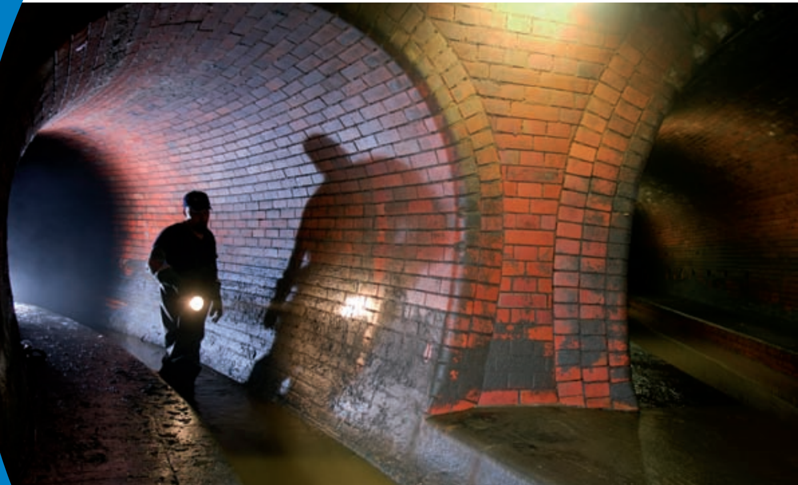
Sewer inspection of the stormwater overflow system at Hohenstaufenstraße
