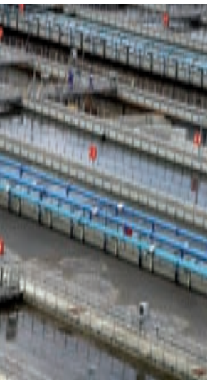
Biological wastewater treatment
