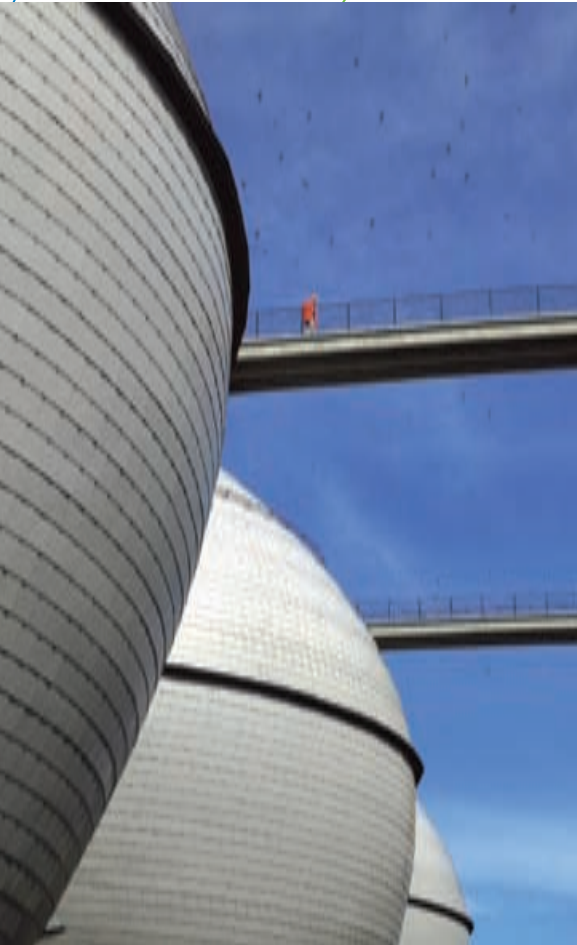
Digestion towers in Ruhleben wastewater treatment plant
