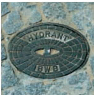
Hydrant (Underground hydrant) on roads or footpaths. Do not block or park on them! The square white sign with a red edge all round is used to indicate hydrants.
