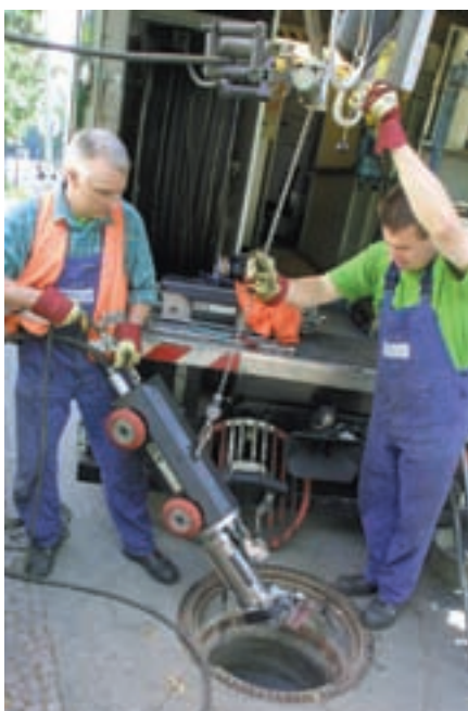
The sewer must be cleaned before cameras and repair robots can start work there. A sludge extraction vehicle in use. A repair robot being lowered into a manhole. Works in the sewer are supervised and monitored from the vehicle.
