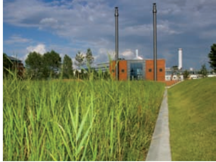
Retention filter at the pumping station Adlershof
