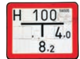
The white sign with red borders indicates the location of a hydrant. The hydrant is located on a 100 mm diameter water pipe. It is located four metres to the right and 8.2 metres in front of the sign.
